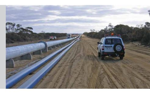
A flexible layflat hose for all types of industrial water supply operations. Offers major cost savings and performance advantages over conventional rigid pipe.
