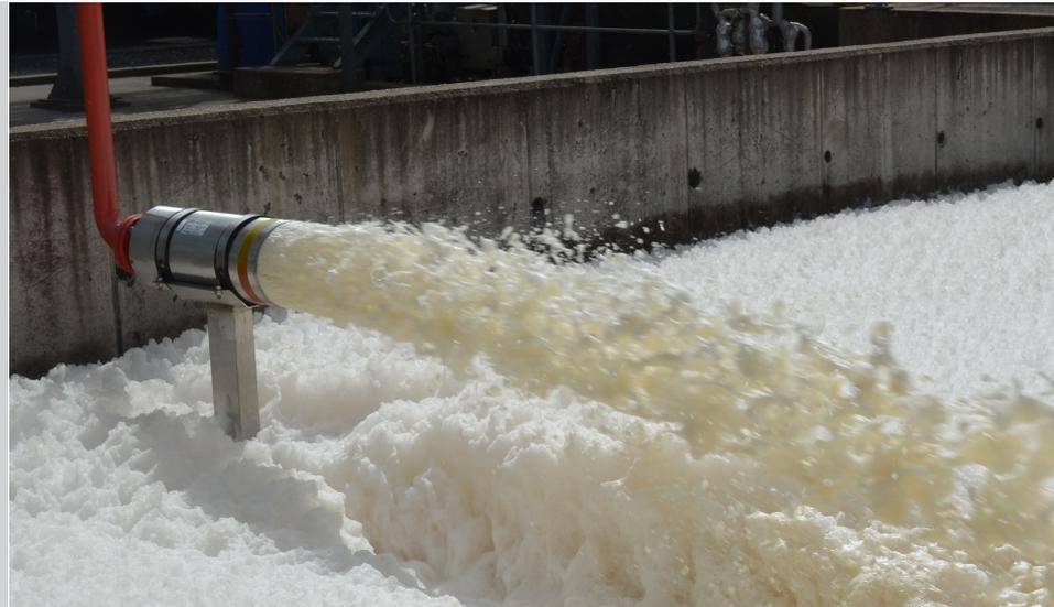
Angus Medium Expansion (MEX) Bund Pourers are designed for fire protection systems and vapour suppression on bunded or diked areas surrounding flammable liquid or toxic chemical storage tanks. They are also suited for other applications requiring large volumes of free flowing foam eg. process areas, warehousing and storage protection.
