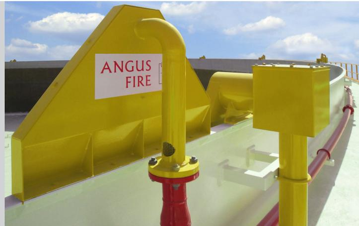
Angus Rimseal Foam Equipment is used for the protection of vertical open top floating roof (OTFR) storage tanks and comprises two elements - the Rimseal Foam Generator (RFG) which produces expanded foam when supplied with foam solution and the Rimseal Foam Pourer (RFP) which delivers the foam gently into the rimseal area.
