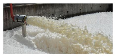
Medium Expansion Bund Pourers are designed for fire protection systems and vapour suppression on bunded or diked areas surrounding flammable liquid or toxic chemical storage tanks.
